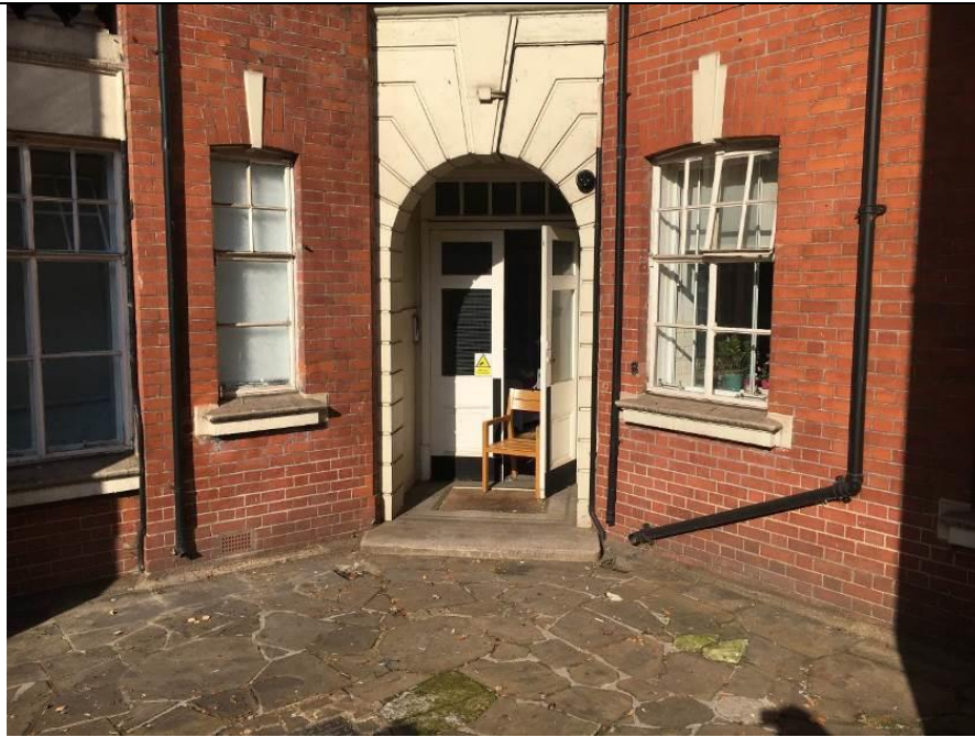
Existing Entrance Doors
